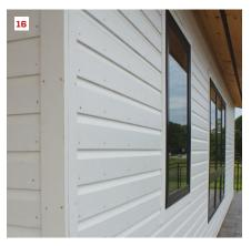
Dutch-lap siding was face-nailed with 8d SS ring-shank nails (heads flush with siding) and installed tight against trim; gapping wasn't required (cut ends don't need priming) (12). Large penetrations were blocked with Boral; head trim was run over jamb trim (13), similar to window (14). Approved filler was used for holes (15). Nails were installed 14 inches o.c. along snapped lines (16).
