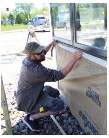
Head and jamb window flanges were taped to the sheathing with Zip flashing tape, then a drainable WRB was installed (2). Metal drip cap and Siga Rissan and Fentrim tapes folded onto the sills' frames (3) were incorporated into the drainable WRB.
