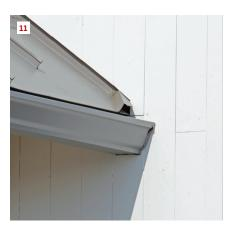
Due to wind, the HydroGap WRB was installed vertically on the north elevation as the siding was installed. The author nailed by hand near windows to avoid damage to underlying flanges and flashings (9). At the stair tower (10), the siding was installed with a 1-inch gap between the roofing and bottom edge of siding; note the kick-out flashing formed into the roofing pan (11).
