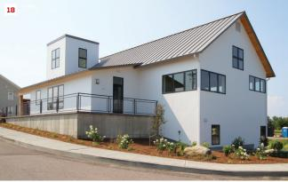
Vertical siding lapped over a fiberglass-reinforced plastic protection barrier at grade. Snapped lines helped line up 16-inch-o.c. face-nailing (17). Hole filler and raw Boral were spot painted (gaps were sealed with urethane-based, paintable caulk), followed by a finish coat of Sherwin Williams Resilience (two coats of paint had been applied to the siding offsite prior to delivery) (18).
