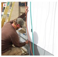
Vertical seams were cut at 30-degree angles (a quality dust mask was a must while cutting) (4). The siding was installed with 2-inch-long ACQ staples 8 to 10 inches on-center, blind-nailed along the sides (6). Joints were face-nailed with 8d stainless steel ring-shank nails (5). Jigsaws and drills with Forstner bits (7) were used to cut the siding around penetrations (8).
