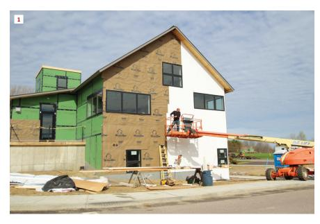
The library was built to be highly durable with 2x8-framed walls sheathed with ½-inch OSB and 2-inch Zip System R-Sheathing (with dense-pack cellulose). Wide windows reduced the number of long grade-to-soffit runs of vertical siding (1).
