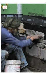
The blend of ledgestone and slightly larger ashlar stone comes with a nominal thickness of  $1\frac{1}{2}$  inches. After trimming each stone to fit, the mason applies mortar to the bare concrete. He then butters the back of the stone (7) and presses it into place (8). The crew uses the same process to apply stone to the scratch-coated areas (9, 10).
