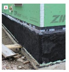
Thin concrete block raises the stone shelf cast into the foundation closer to grade (1). Flashing tape protects the bottom of the sheathing behind the metal lath (2). The black scratch coat provides a dark background for the "dry-laid" stone (3).
